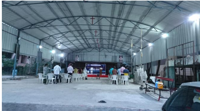
Hyderabad YMCA Temporary Building
